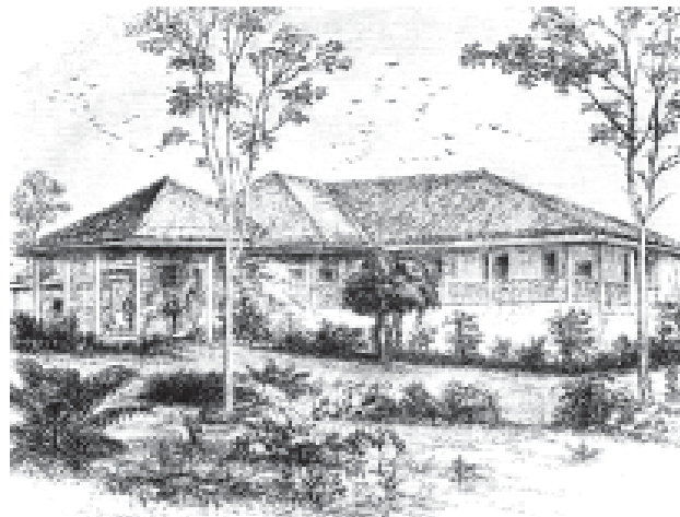
Fig. 12.23 A bungalow in Bombay, nineteenth century
