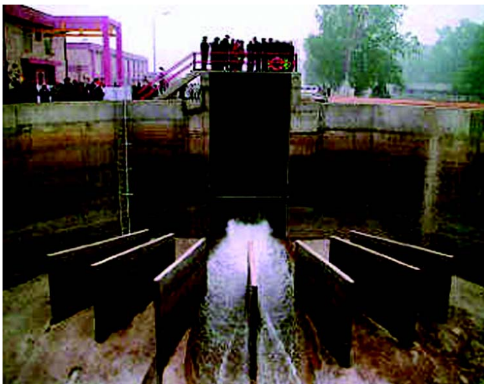
Fig. 18.10 : Water treatment plant
